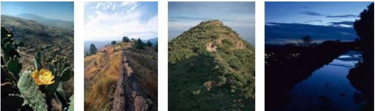
Fig. 9. Slopes Stone canal The collector The perimeter road
